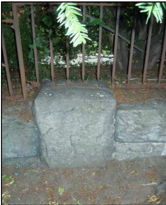
Rough cut granite used on sides and back
