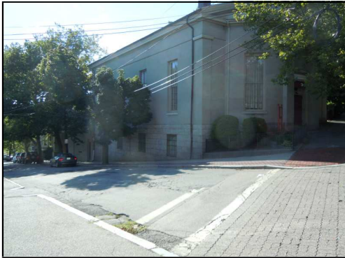
From front slope south, not changed
