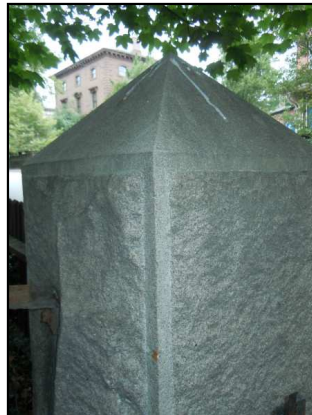
Front corner stone with dressed or finished edges
