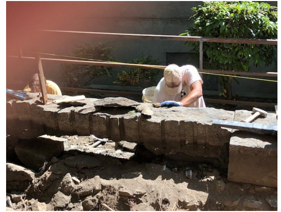
Masons repairing the stone wall this fall.
