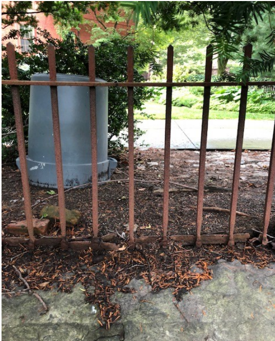
Badly rusted fence on north side
