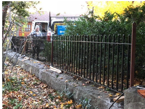
Repaired south wall with original fence back.
